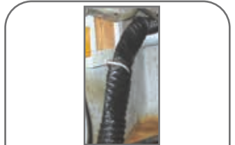
Crushed vent ducting, will impede proper and safe venting of fumes. Replace damaged duct
